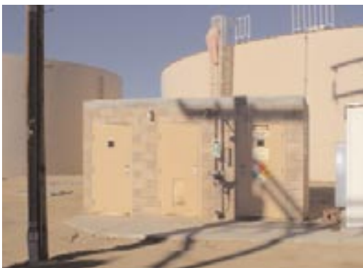
Existing chlorination station at one of the District's well fields.
