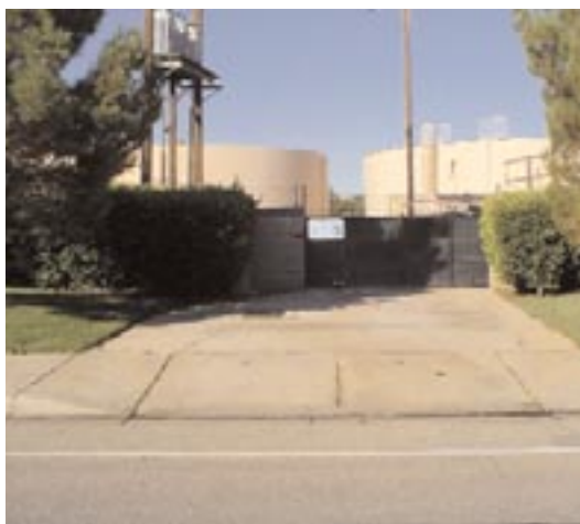
Existing security fence around one of the District's facilities.
